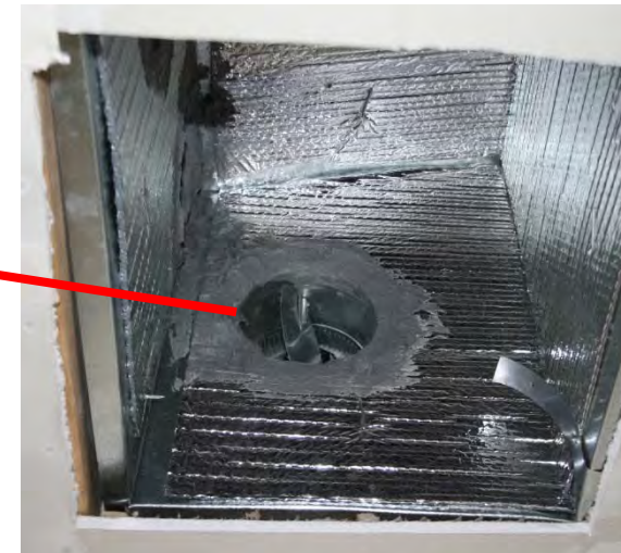
An outside air intake inside a return plenum using a motorized damper.
